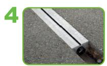
Level out the cones. Be careful to leave enough space without flanking, when a final covering (tiles, blockpaving, etc...) is necessary.
