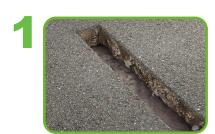
Realize the excavation according to the dimensions required in the project. The dimension will be on the diameter of the required pipe.
