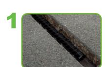
After having carried out the excavation as per Phase 1 and 2, insert a suitably bent "U" shaped welded mesh panel resting the part open on the bottom of the excavation.
