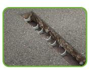
Lay the EPS supports on the bottom of the excavation site suitably compacted and leveled.
