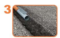
Lay the collection element on the laying bed. Link up the drainage pipes to the sewerage.
