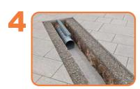
Lay the the collection elements on the laying bed. Link up the drainage pipes to the sewerage.
